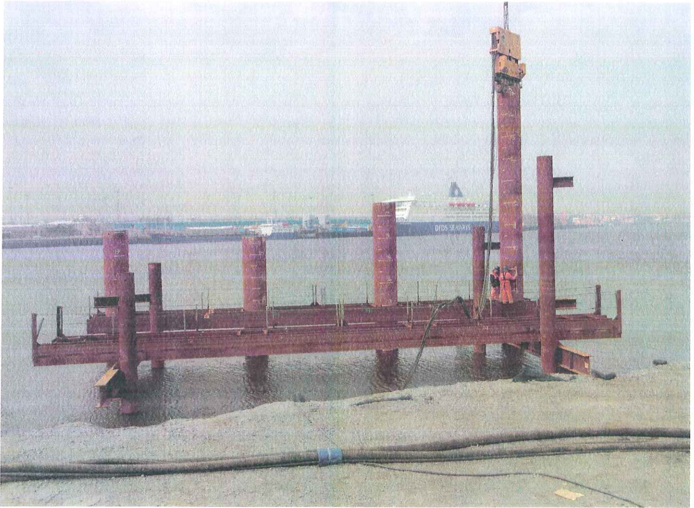
Typical piling frame
