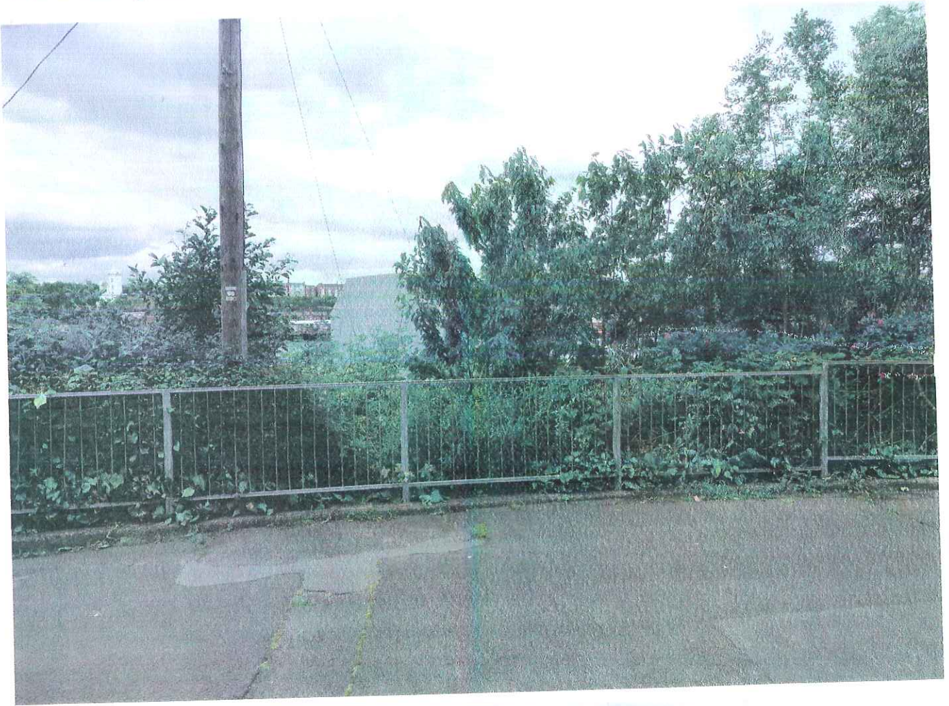
View of existing boat shed from Greens Place
